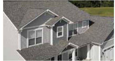
ROOFING AND VENTILATION
